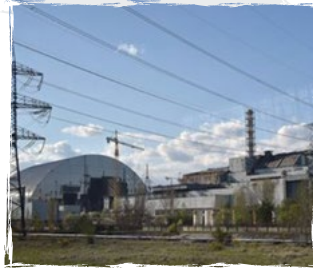
PANAROMA VIEW OF THE CHERNOBYL POWER PLANT
