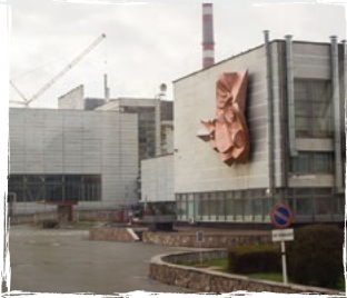
MAIN ENTRANCE TO THE POWER PLANT
