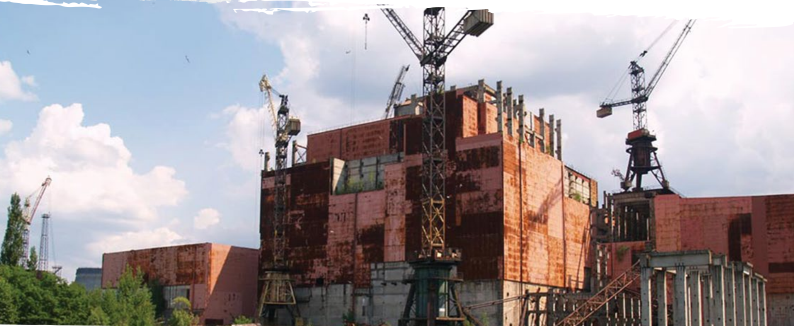
UNFINISHED REACTOR 5 AND 6
