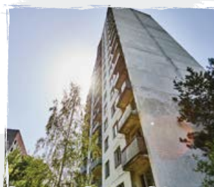
HIGHRISE BUILDING WITH USSR EMBLEM
